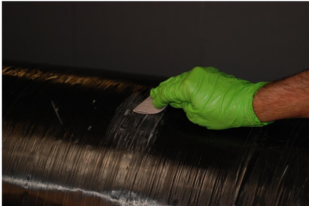
▲ **Optional:** When the epoxy is fully cured and dried, sand the surface again.
