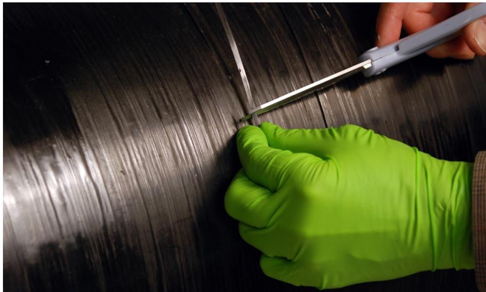
▲ Trim off delaminated fiber at the widest and deepest point. **Note:** Only delamination of the outer hoop wrapping may be repaired. The width of the delamination may not be any wider than the original area of damage from cuts, gouges or abrasion (see Section 6.6, above).
