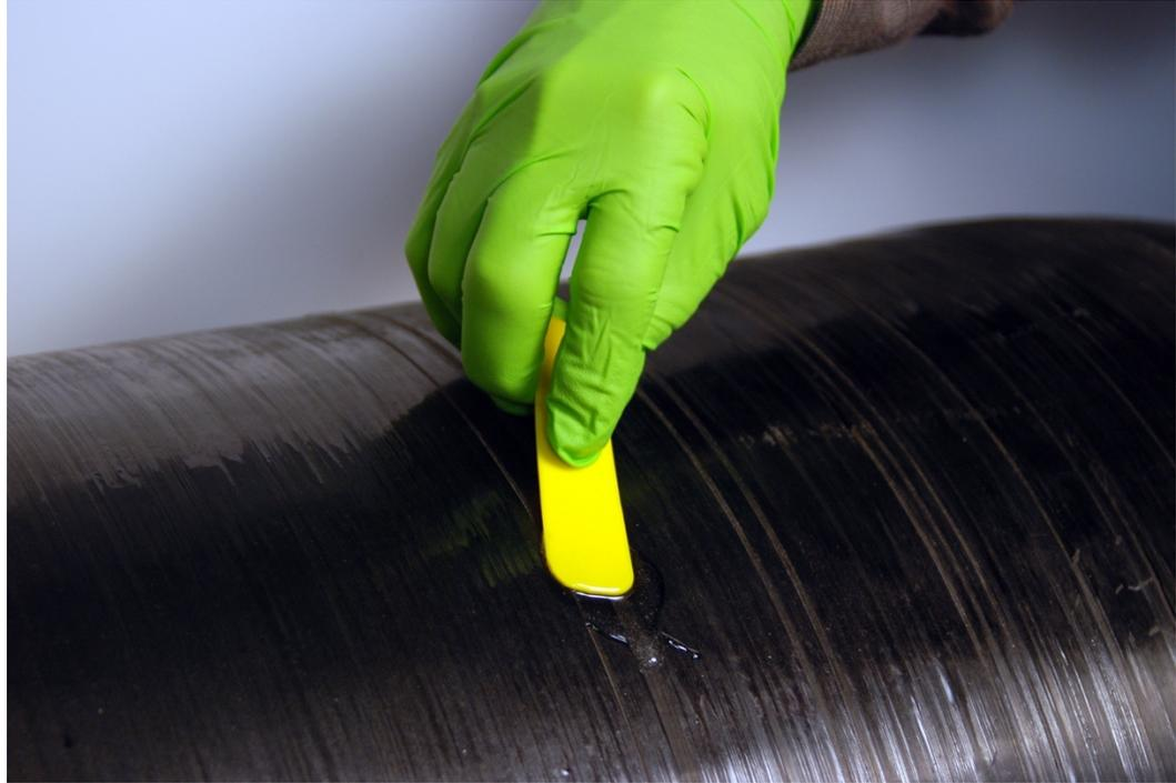
▲ Follow the procedures shown previously above to mix epoxy resin. Generously apply resin to the gap left when delaminated fiber was removed from the outer hoop-wrapping.
