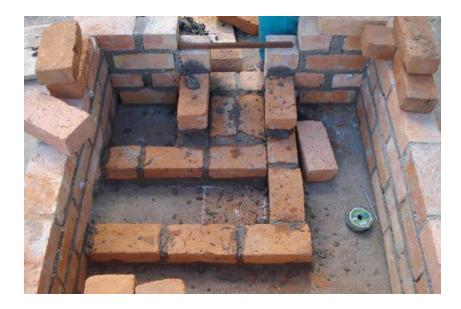
FIGURE 3 The firewood inlet being built extending over the combustion chamber and the Air inlet being built over this<sup>xxvi</sup>
