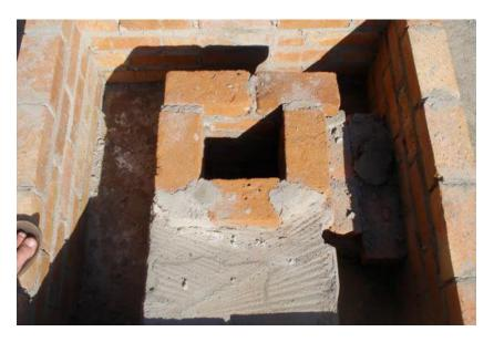
FIGURE 4 The combustion chamber built with a supporting wall
