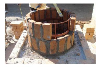
FIGURE 6 Insulating bricks laid around the pot skirt stabilizer. Space is left in the second line to insert the chimney
